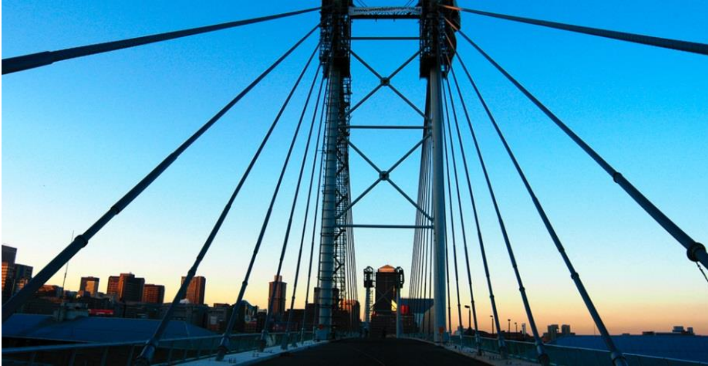
Nelson Mandela Bridge
